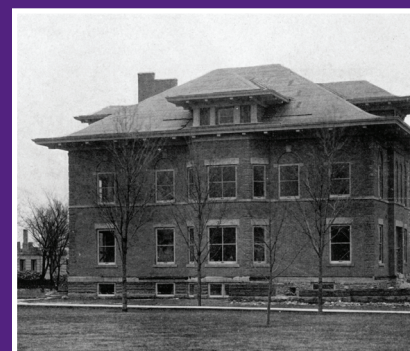
The current President's House under construction in 1909.
